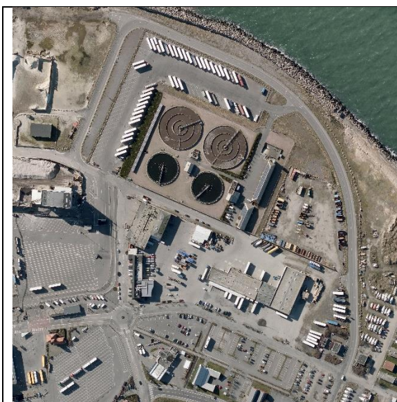
Figure 9 Rønne Waste water treatment plant
